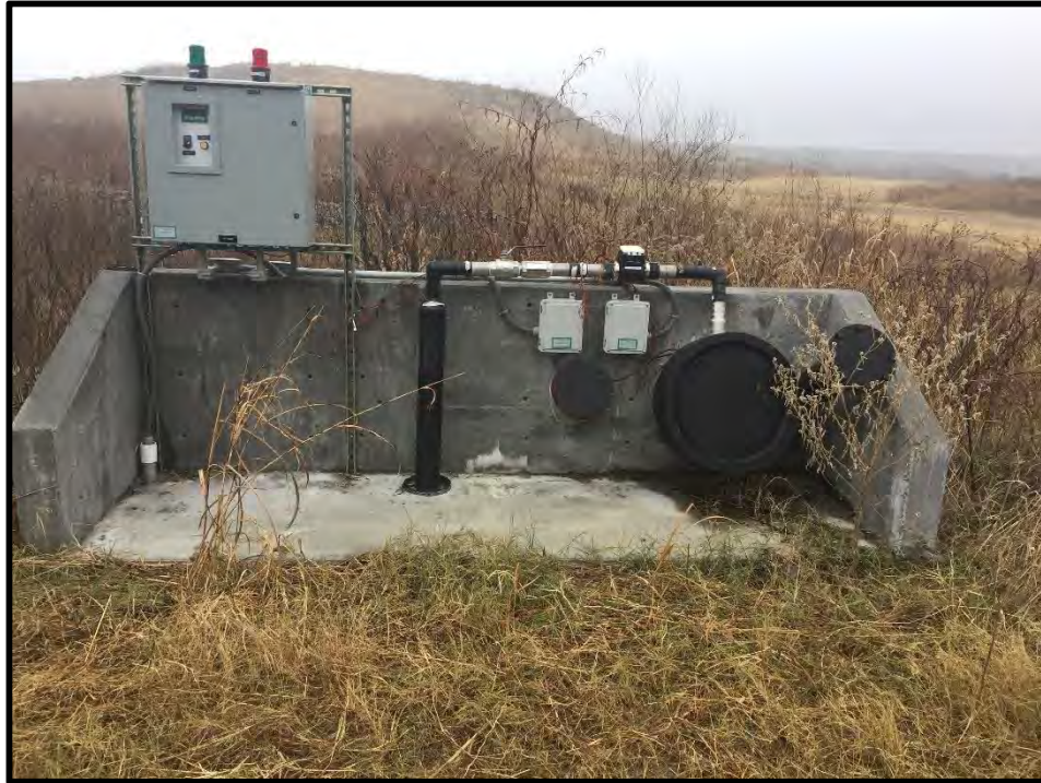
5. Leachate pumping system on the southeast corner of Cell 4.
