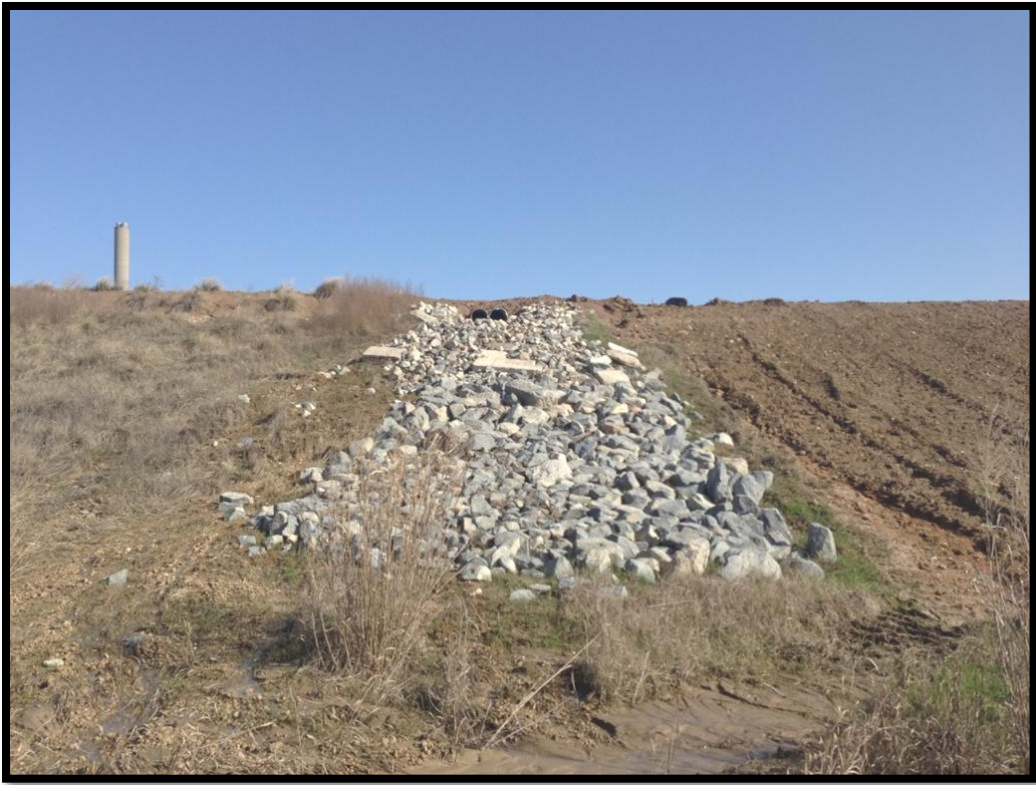
Photo 7: Riprap lined letdown, southwest of Cell 3
